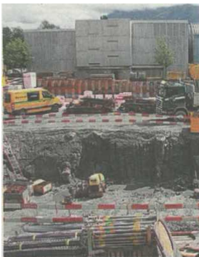
Current construction site.
